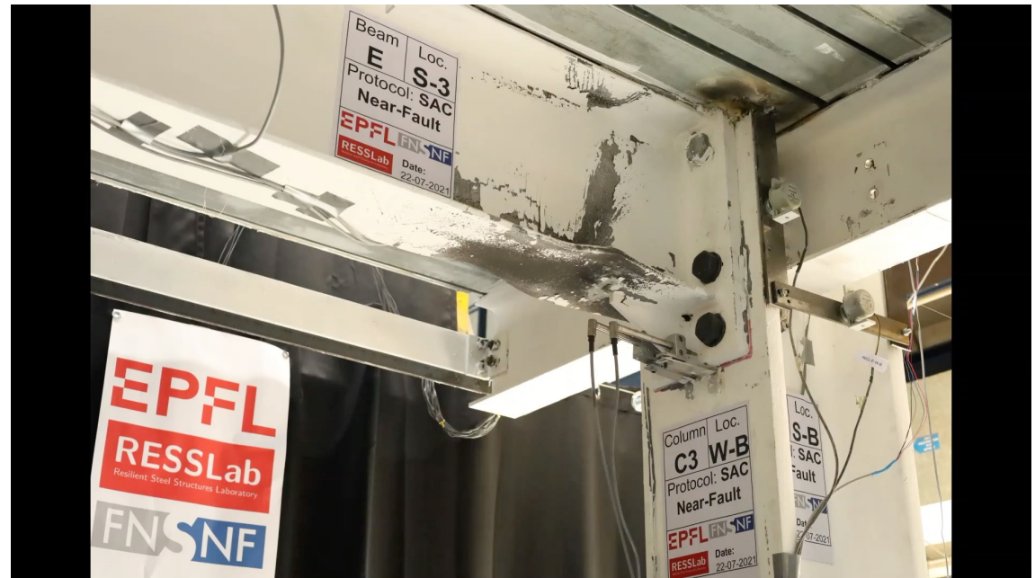
East beam: Exterior Joint
